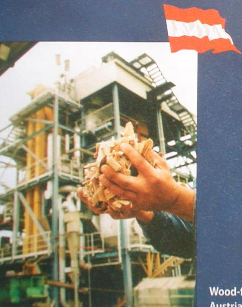
By means of injection pipelines the waste wood (swarf and sawdust) from the neighbouring parquet factory is injected directly into the silo, from where it is taken automatically for combustion in the heating plant. To the right, a 27 kW<sub>p</sub> PV system can be seen that feeds electricity into the grid.
